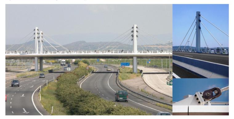
The new link motorway between the southern Valencian distributor and the A-7 motorway which by-passes Valencia, shall need to cross the latter and its service roads set at a 45° skew and without need of supports on the central reservation of the A-7 so allowing for possible future widening of the aforementioned. The connection at the junction area shall have two carriageways, one 7.0m wide and the other 4.0m, two 2.5m hard shoulders and a 3.0m wide central reservation.
